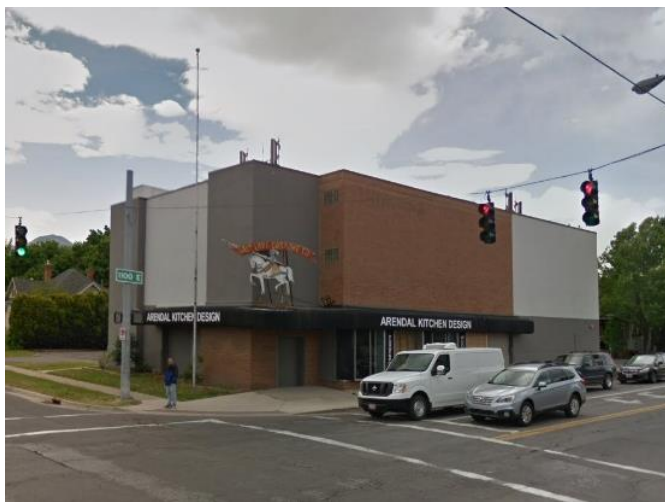
View of existing building looking south east from 1100 E.
