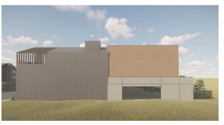
This building elevation is 0'-0" from the adjacent property line, and will be a fire-rated wall with no openings. Additional detailing of the coffee shop trellis wil soften this elevation, along with minor steps between building material elements
